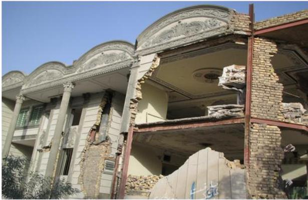
**Fig.2.** traversal throwing of infilled in bam earthquake in 1382. (Iran)
